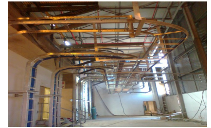
Cable Tray Installation on Site
